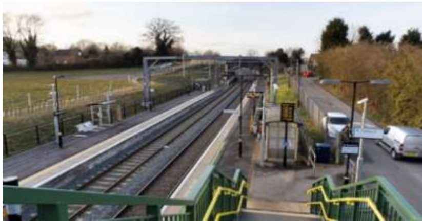
Fig 57. Alvechurch new rail station completed 2015
