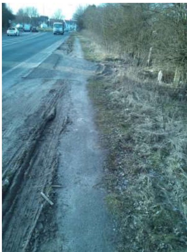
Fig 63. Results of Large Goods Vehicles parking on highway footways, A441
